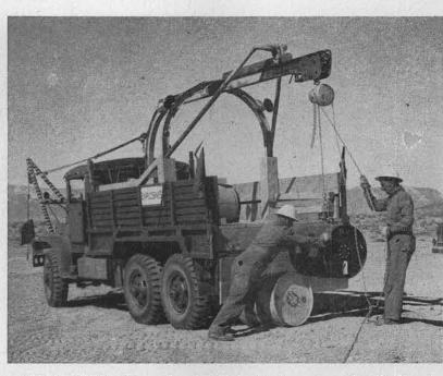
EXPLOSIVES-600 pounds of TNT in the form of an obsolete Naval depth charge are swung into position by Donadieu "Frenchie" Sonnier. 1932, as Jerry Ward, Field Test high explosives man, 5212, mans the hoist. The HE is detonated before a nuclear explosion to predict shock
